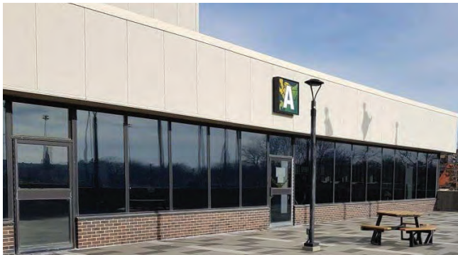
Upgrade of the library balcony.
