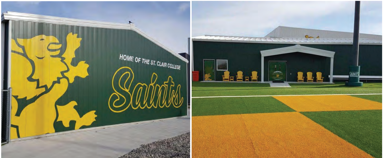
The construction of the Saints Football Field House.
