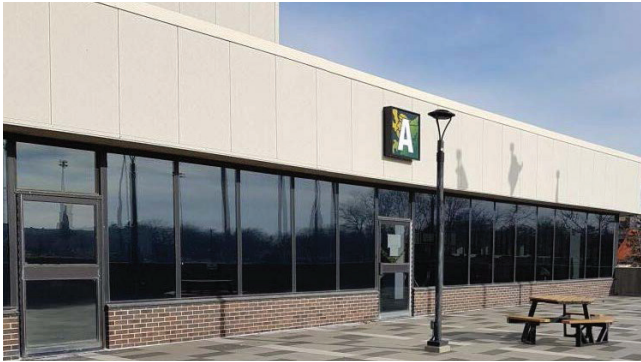
Upgrade of the library balcony.
