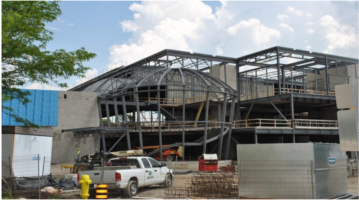
Figure 5. The Windsor Campus Sportplex under construction.
